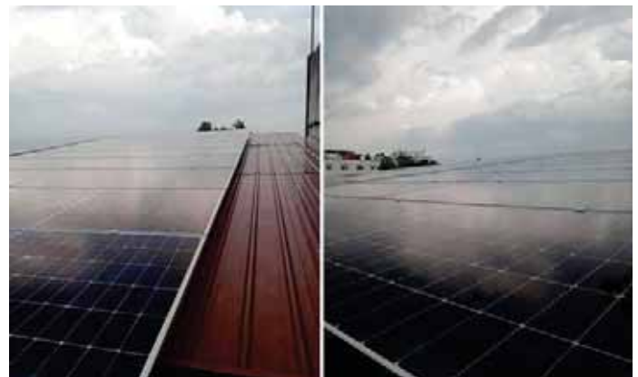
Solar Rooftop System installation at Horana Branch underway
